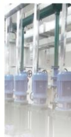
PUMPING STATION 泵站
